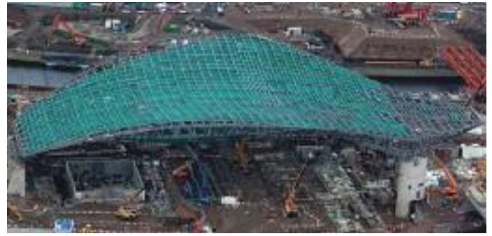
Aquatic Centre construction
