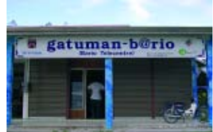
Tele Centre with photovoltaic-technology Photo courtesy Mike Khaw
