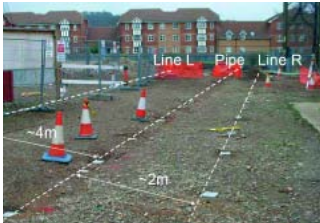
Pipeline and BOTDR positions at Chingford
